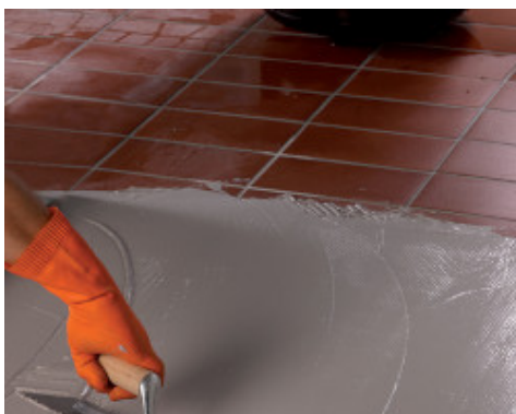
Applying a second layer of Monolastic on Mapeket 150
