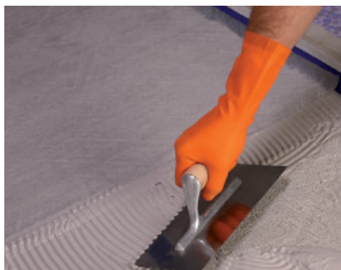
Applying a first layer of Monolastic welded with Mapetex Sel on a new screed
