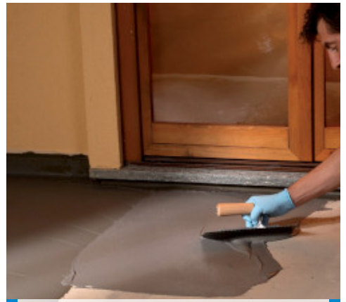
Waterproofing of terraces by trowel
