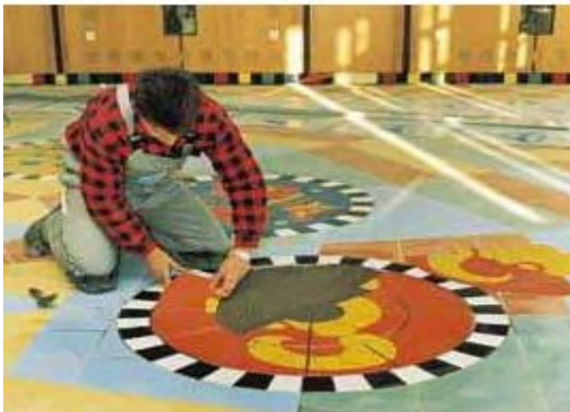
Secure laying of tiles with MasterTile FLX 23
