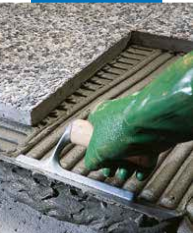
External installation of relief terrazzo "graniglie" tiles
