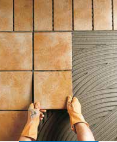
External installation of klinker tiles
