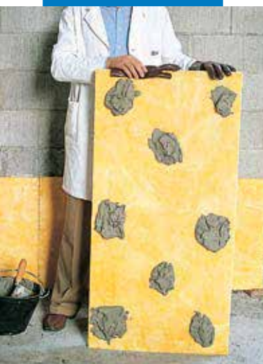
Spot-bonding insulating panels on untreated wall
