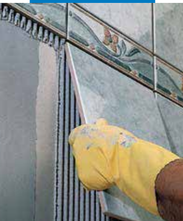
Installation of single-fired tile on wall render
