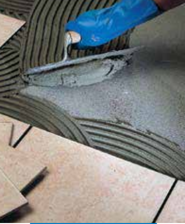
Installation of single-fired tile on floor
