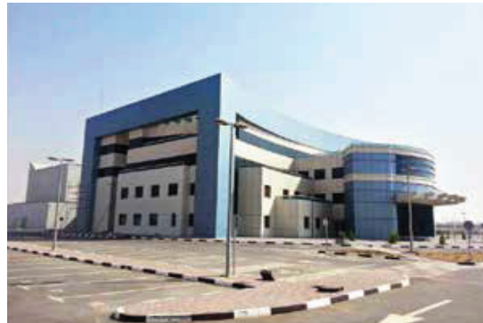
Al Barsha Police Station Abu Dhabi
