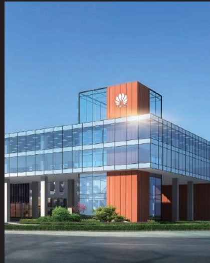
Huawei Cloud Computing Center
