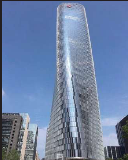
Bank of China Data Center
