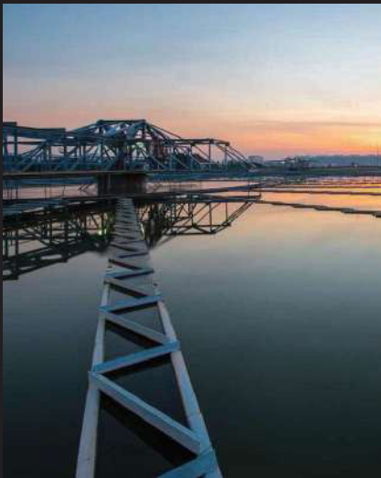
ABU DHABI Water Supply Project
