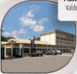
VIR Warehouse Valduggia (VC) Italy
